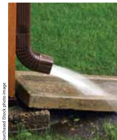
Downspout directed into the yard.
